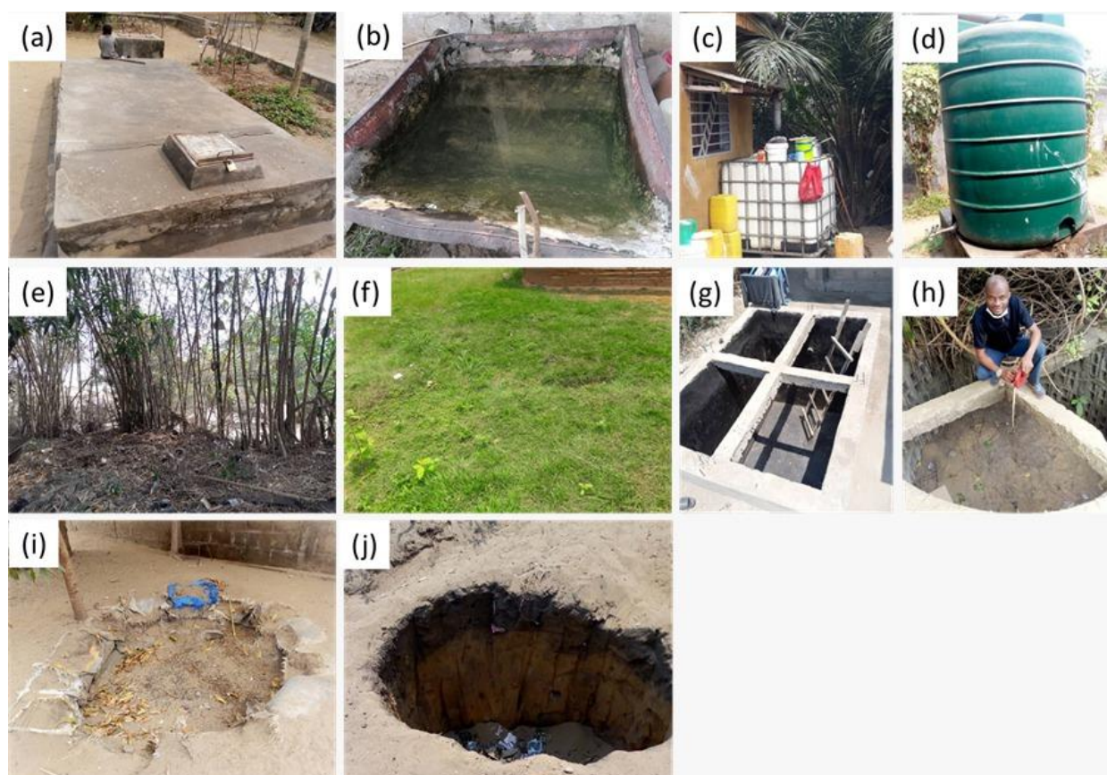
Fig. 3: Examples of runoff water retention measures observed for the collection, storage, and infiltration of rainwater. a and g: Sealed underground masonry tanks; b: Underground metal tank; c and d: Plastic rainwater tanks (small and large capacity); e and f: Vegetation enhancing infiltration rates and preventing bottom clogging; h: Soakaway pit with concrete blocks; i and j: Infiltration trenches.
